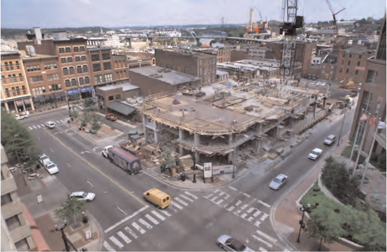
Commercial development was booming not only in the vicinity of suburban shopping malls; there was evidence of it in downtown Nashville too: the Magnetek Building at Third and Commerce.
